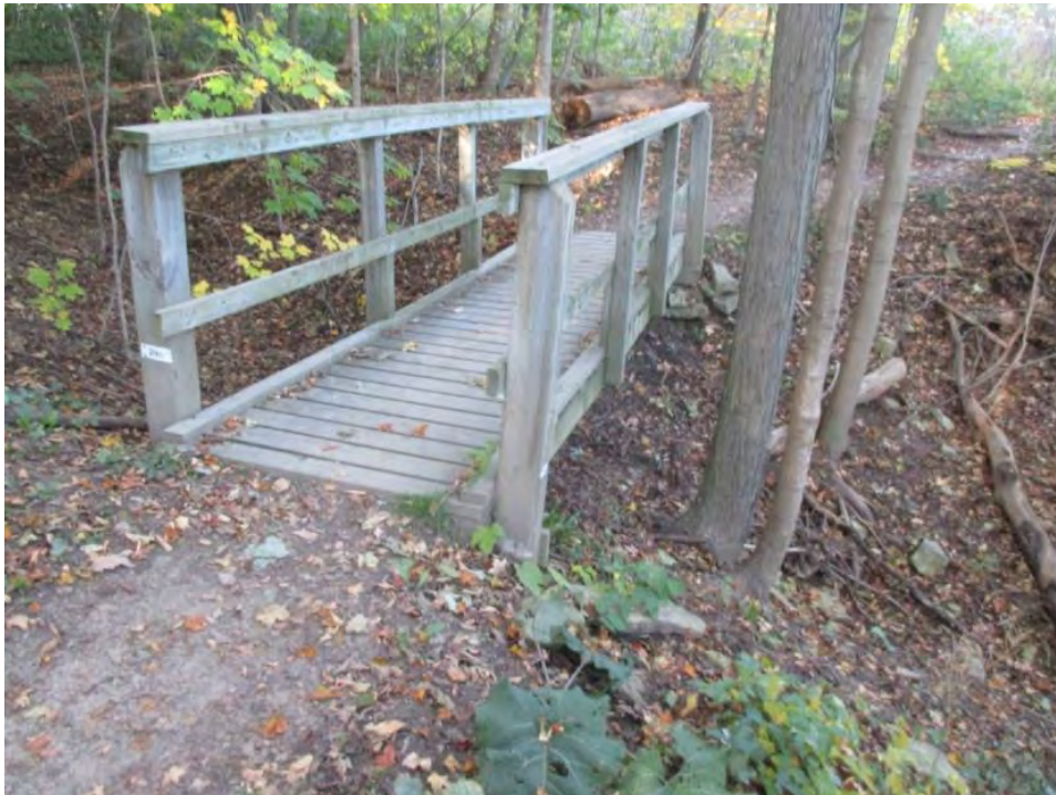
Photograph 23: Wooden bridge along Bruce Trail in Rock Chapel 1.
