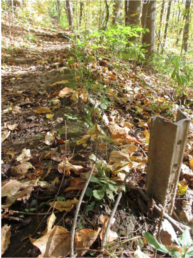
Photograph 10: Cut down signpost is a tripping hazard.
