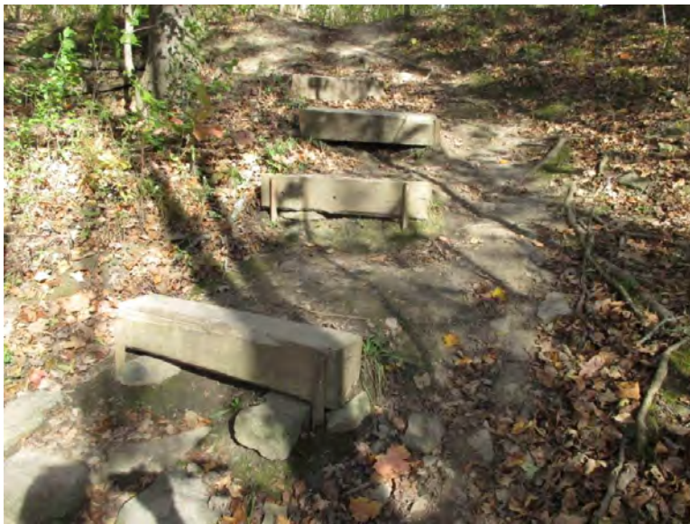
Photograph 3: Trail erosion, unsanctioned cycling activity evidence and failing earthen staircase in Borer's Falls Conservation Area 1.
