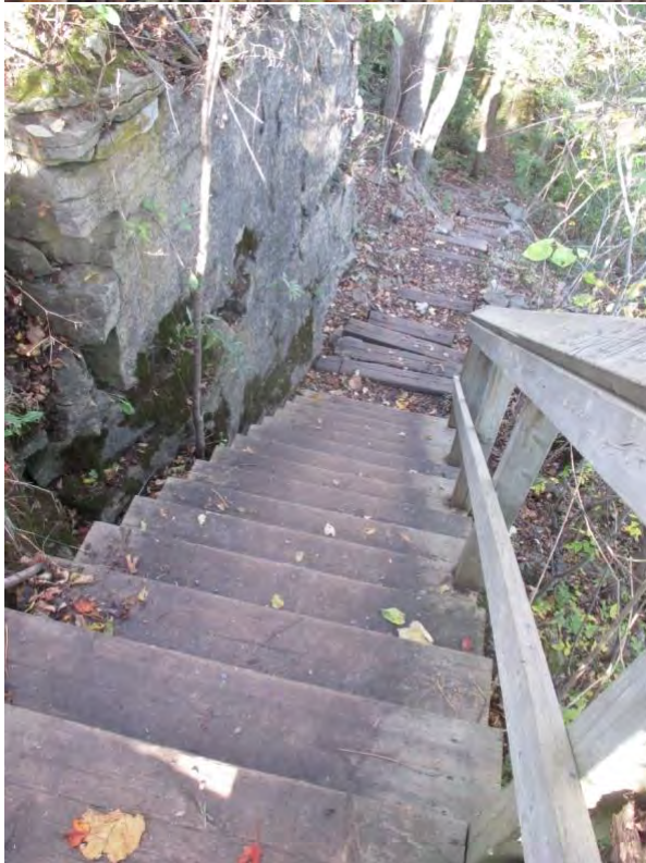
Photograph 13: Series of staircases up the Niagara Escarpment cliff face in Rock Chapel 1.
