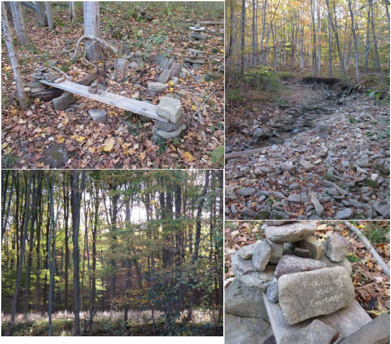
Photograph 29: Unsanctioned trail structures and erosion along Borer's Creek.
