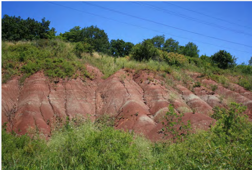
Photograph 2. ‘Badland’ formation following clay extraction for brick making, adjacent to Falcon Creek (Photograph taken by Nigel Finney, Conservation Halton).
